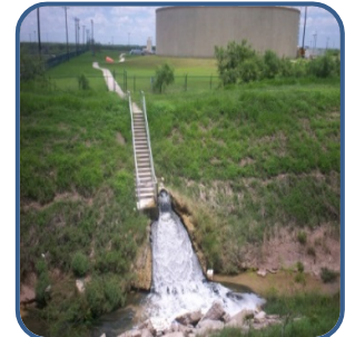
Concentrate Disposal to Drainage Ditch
